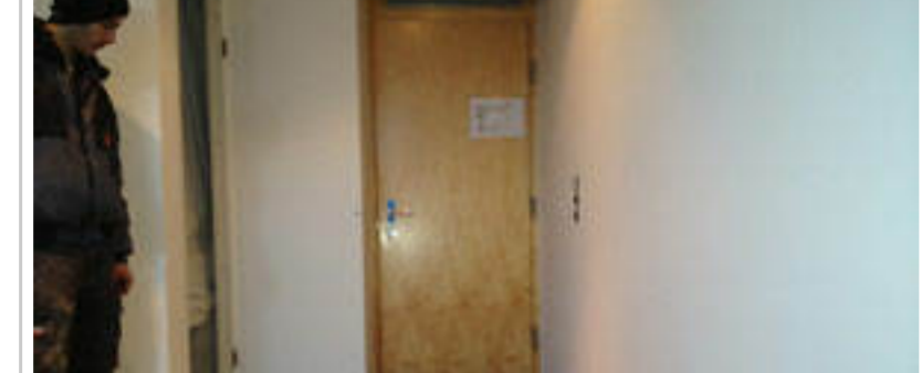
Walls shielded with T98 shielding paint
